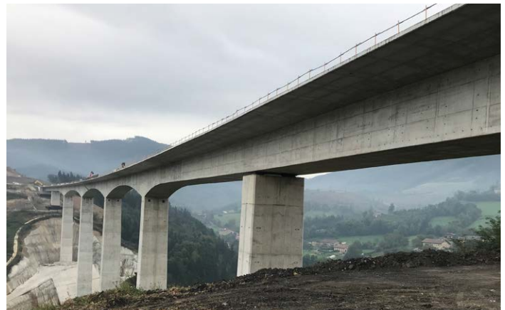
OpenBridge saved 1,000 work hours and mitigated potential costly and time-consuming on-site errors.
